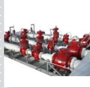
Pressure reducing stations
